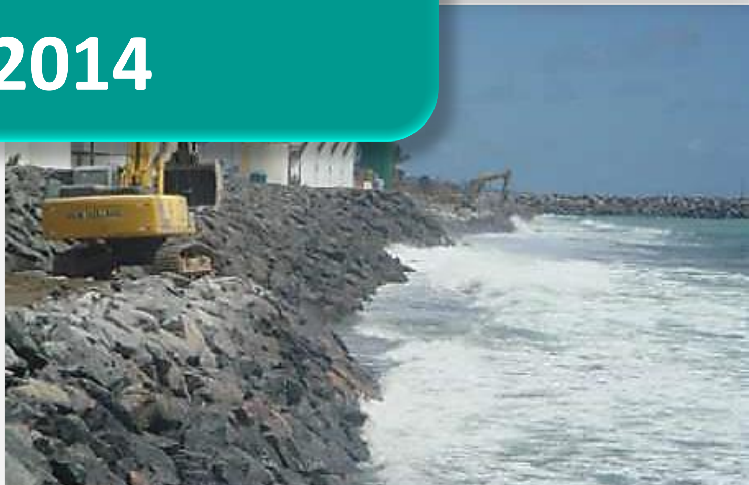
Strengthening of the protection wall
